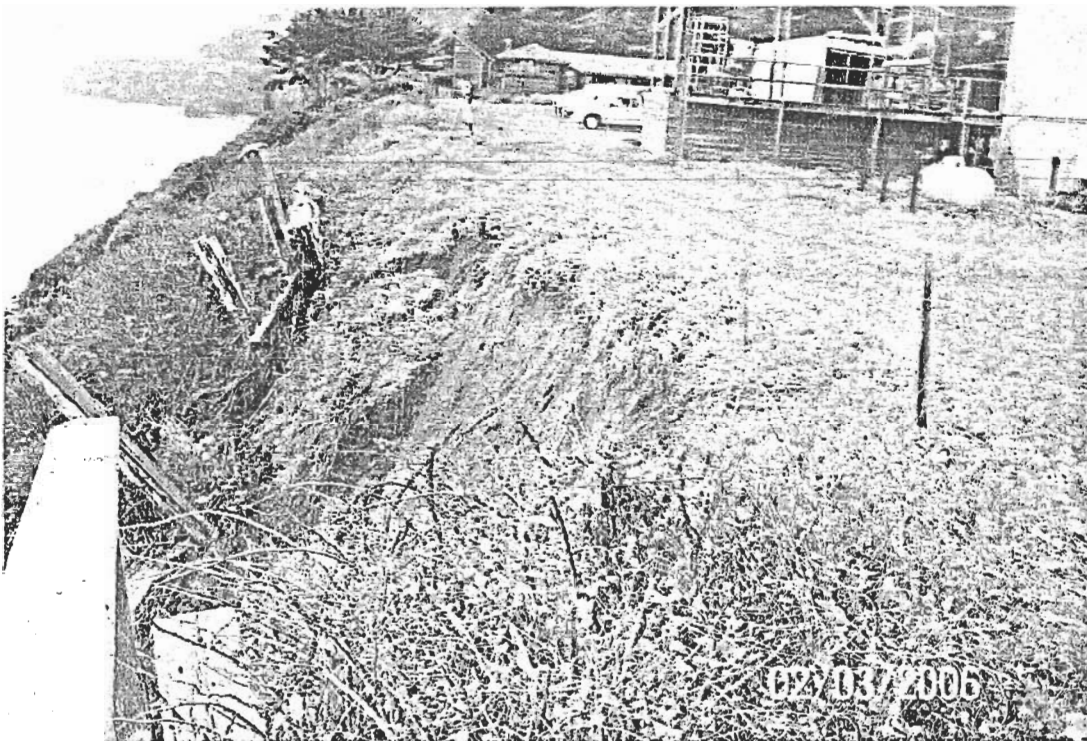
Photo 2. Fill failure
