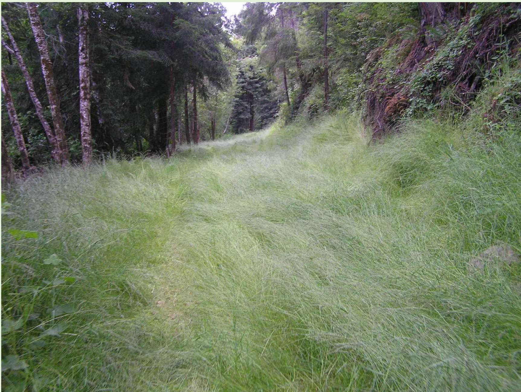
Floodplain haul road erosion control using invasive non-native ryegrass
