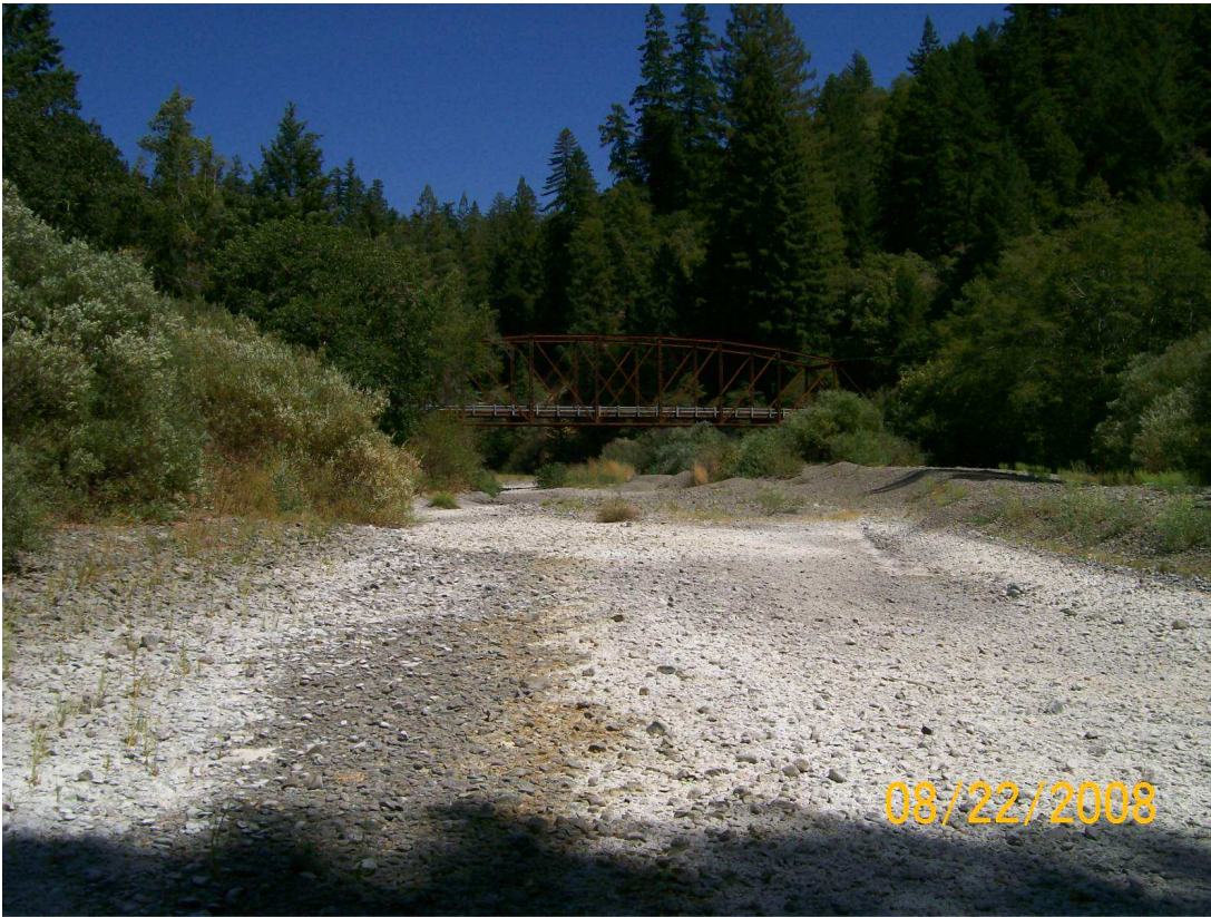
VIEW FROM BELOW BRIDGE(CLARK'S CROSSING)
