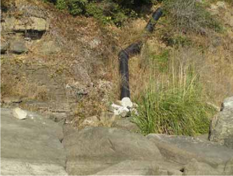
Figure 7. PVC pipe adjacent (west) of project area, apparently unauthorized. Source of discharge is unknown. Cumulative impact of this point source and nonpoint sources of discharges to the lagoon were not addressed at all in the Staff Report. October 1, 2007. Author photo.
