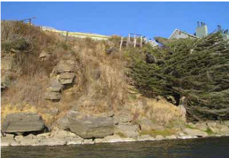
Figure 6. Shallow debris slide of oversteepened, poorly drained past artificial fill, east of proposed retaining wall (separate proposal). Note weed dominance of disturbed sediments. Author photo, October 1, 2007.
