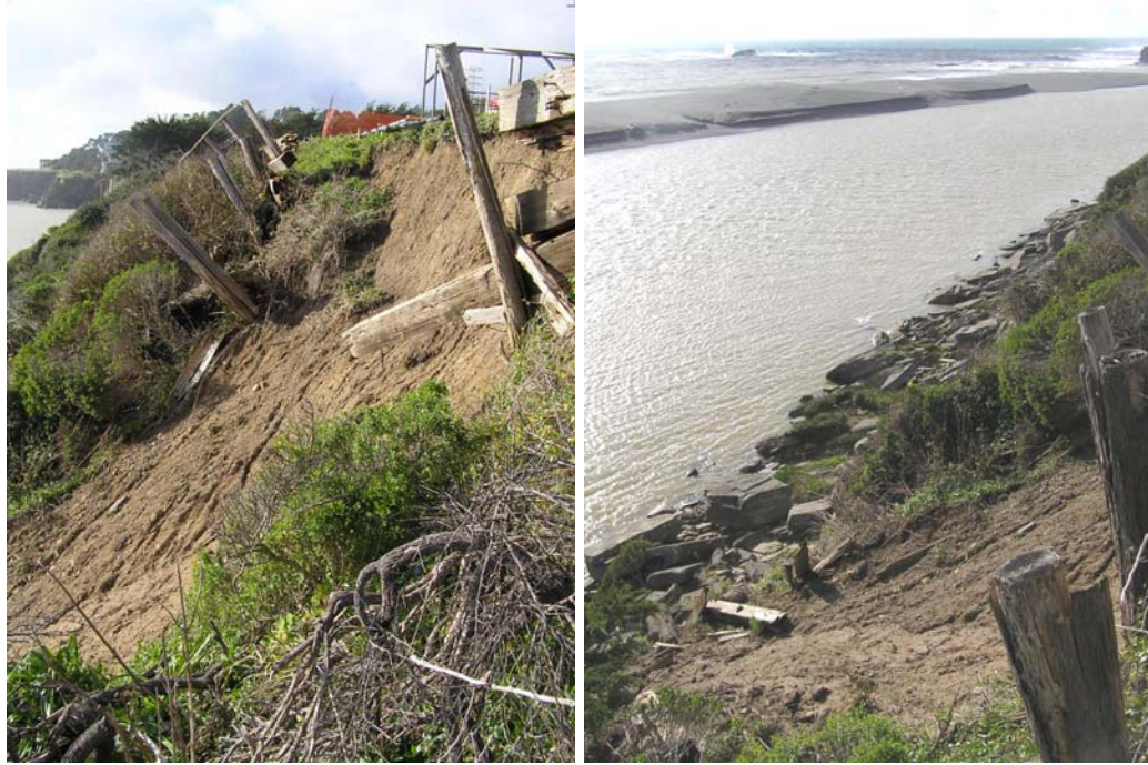
Figure 1. Slope failure (debris flow) behind Surf Supermarket, exposing artificial fill. Note boulder armor beach with marsh pockets at toe of slope. March 17, 2006.
