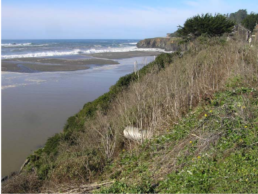
Figure 5. Culvert embedded in artificial fill of project area, under non-native vegetation, discharging above Gualala River lagoon. December 22, 2006.
