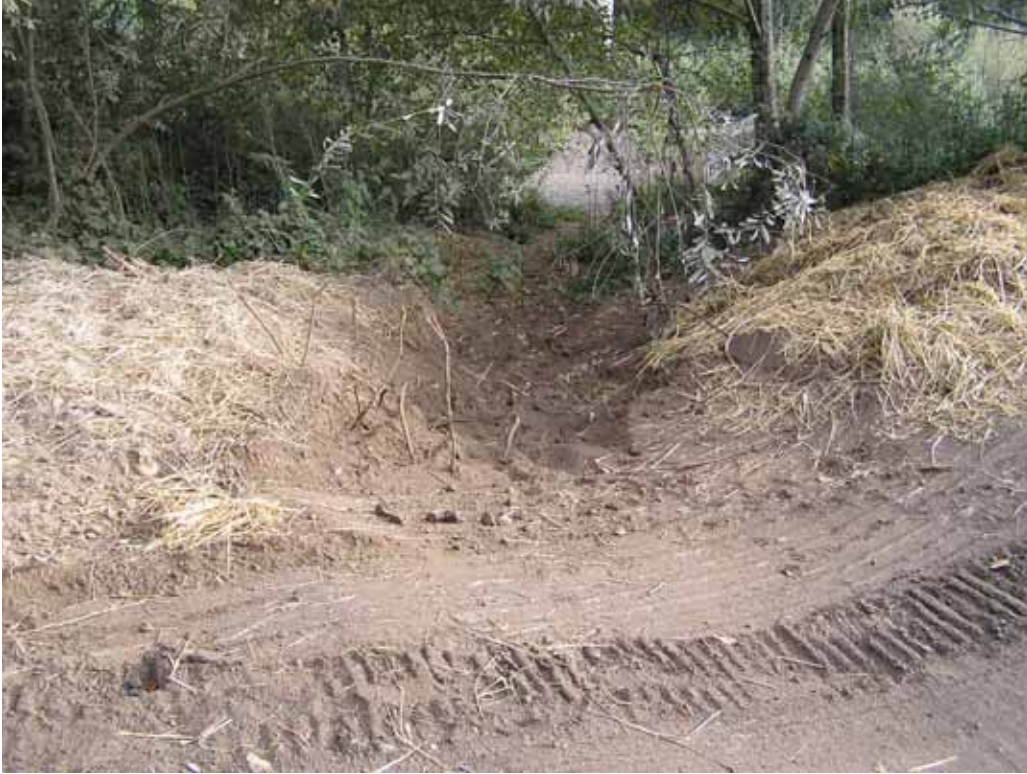
Fig. C-2. New drainage of road and floodplain to river; unconsolidated fine sediment source
