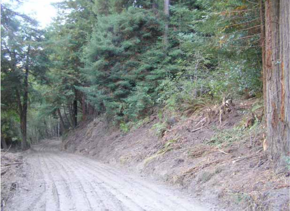
Fig. B-1. Large riparian tree canopy gap on both sides of road, to recent tree removal in riparian zone, including floodplain below road. Steep bank above road is devegetated, exposed soil, unstabilized. Note sediment and slash below road. Logs were apparently removed.
