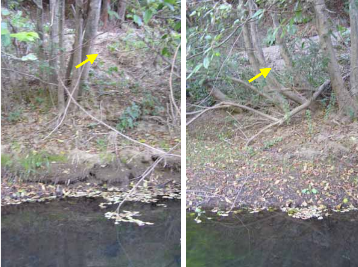
Fig. A-7. Road grading spoils (yellow arrow) deposited over steep bank above channel pool with fish and frogs, flood channel, viewed from channel pool.
