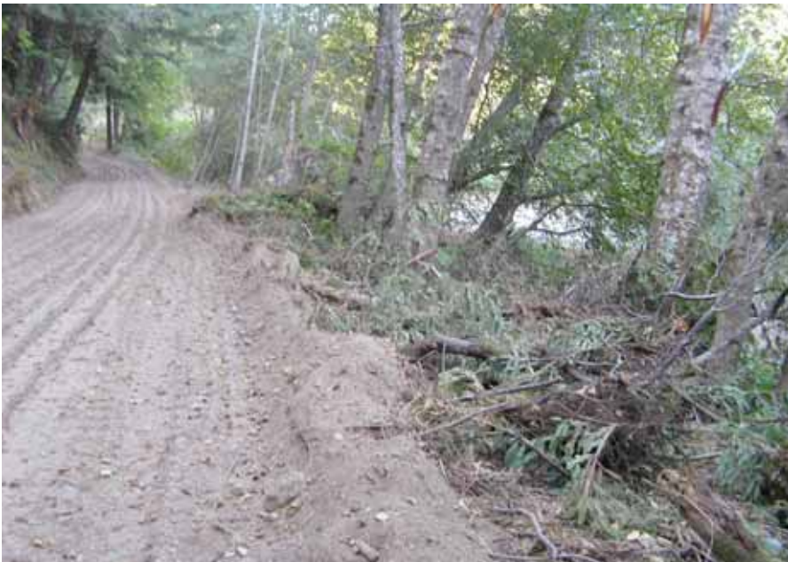
Fig A-3. Slash and loose sediment are deposited at top the widened road in the floodplain riparian zone; road now spills over the formerly vegetated riparian bank. Winter high flow channel bed is directly below. Bank top is below flood elevation, indicated by persistent flood debris in alder branches and silt deposits on road.
