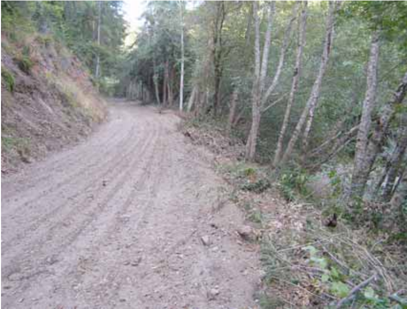
Fig. A-1. Red alder thicket is cut below the widened road edge. Slash, plant debris and loose graded silt is deposited over the bank, above the active winter overflow channel of the Wheatfield fork (right). Note the canopy gap through the mature riparian zone on both sides of road, leaving only alders below grading/”brush clearing” line to provide streamside canopy cover and shade. Road bank upslope is partially
