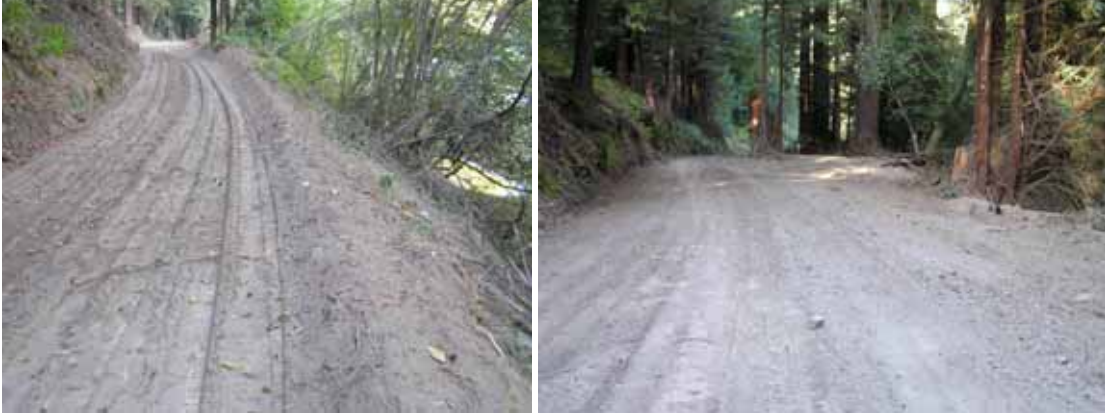
Fig. A-5. Single and double road widths. (a) Loose silt is deposited over road edge and into riparian woodland and forest. Side-cast graded silt spills over steep channel bank. Road here represents a single truck width, the approximate original width. Contrast with (b), widened road segment in right photo, almost double the width, extending into riparian forest. Note tree stumps (background) with fresh wood exposed.
